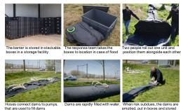
Figure 1: How to operate the technology
